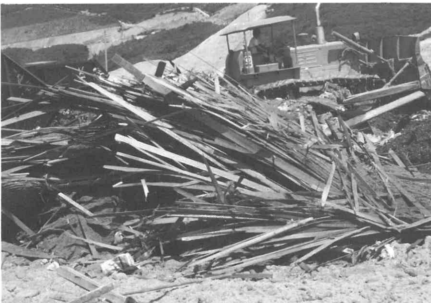
Waste timber buried at controlled tips in Hong Kong, ignoring its calorific value.
